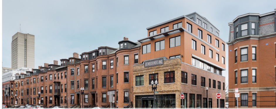
Parmelee Street Apartments - Boston MA Stack+Co. Architecture, Construction
